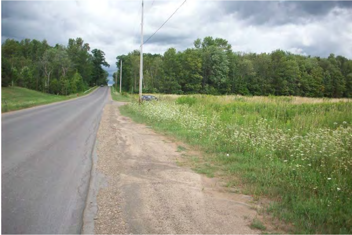
Photograph 1: A small parking area (where car is parked above) was created by the Oswego County Highway Department from asphalt millings to provide parking for snowmobilers.
