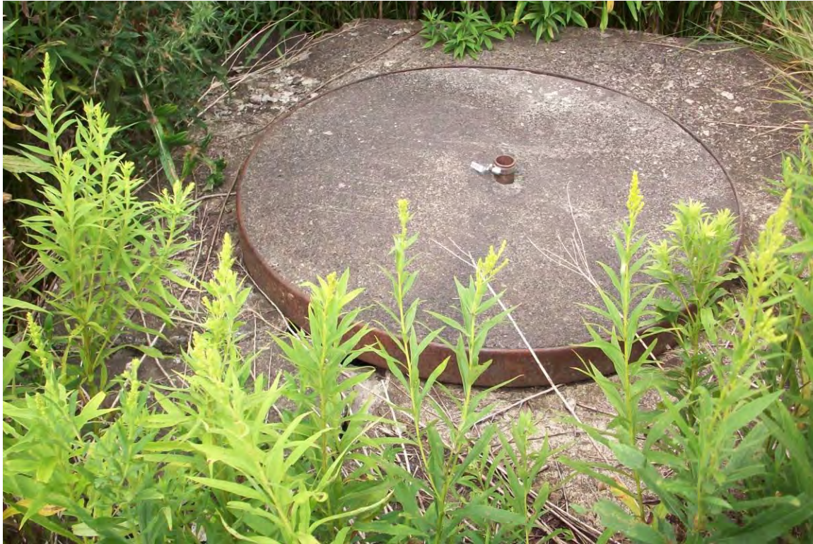
Photograph 105: A concrete manhole was observed on the western side of the site; it is reportedly related to a former well house.
