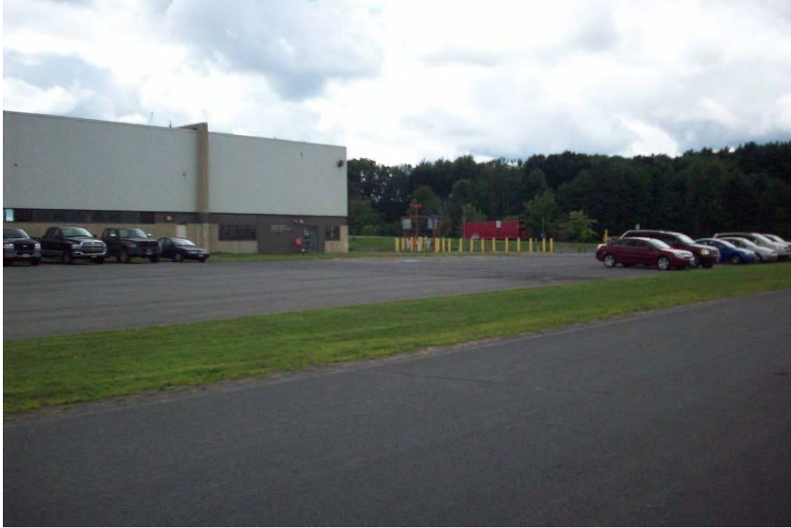
Photograph 21: The Oswego County Highway Department Pulaski Garage is located south of the site across Centerville Road. Petroleum bulk storage was observed in the paved parking area.
