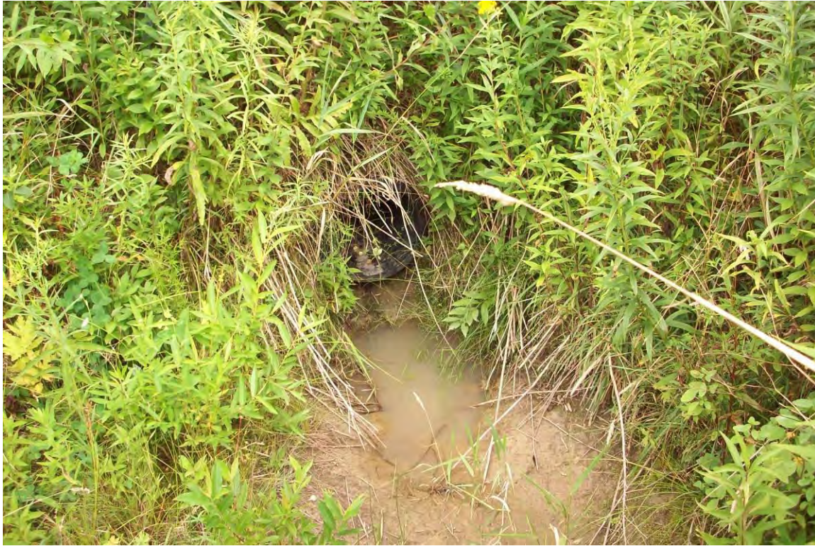
Photograph 7: Ponded water was observed near one of the culverts at the northern end of the site. Water was not flowing during the site reconnaissance.
