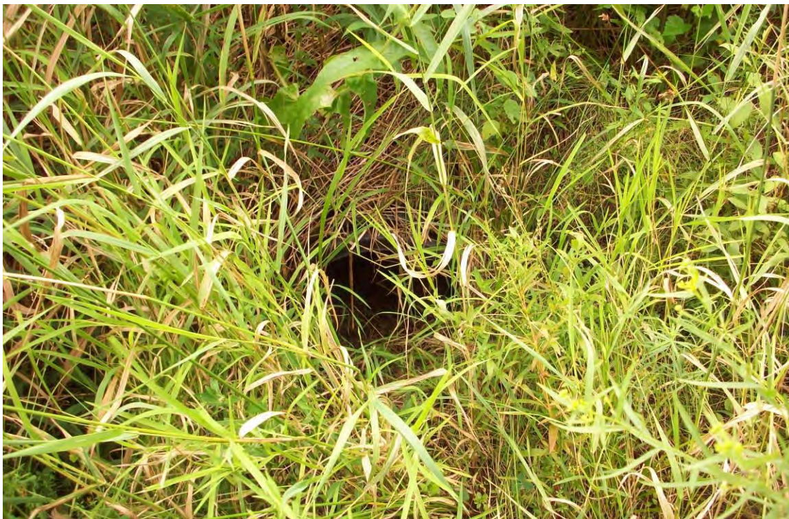
Photograph 6: Culverts were observed in each of the drainages running southerly. They appear to drain the wooded area north of the site onto the target property.
