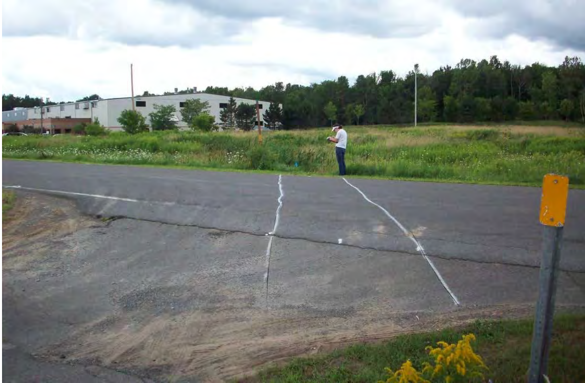
Photograph 11: View facing north of the culverts connecting catch basins across Centerville Road to the ditch shown in Photograph 10.
